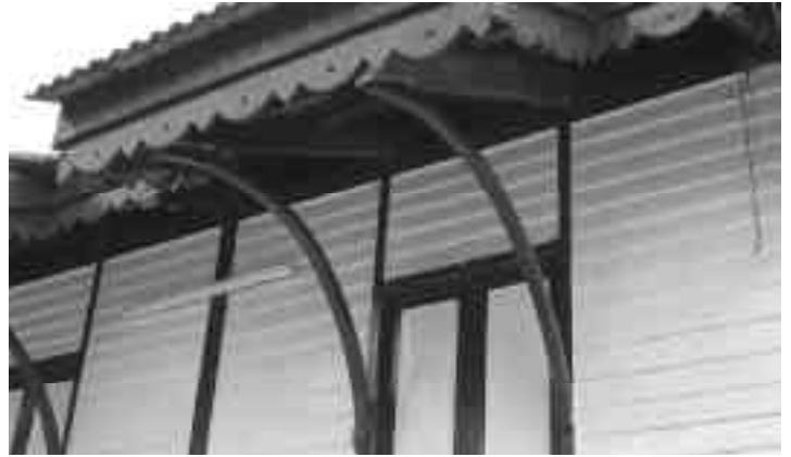
Detail of brackets supporting the roof.
