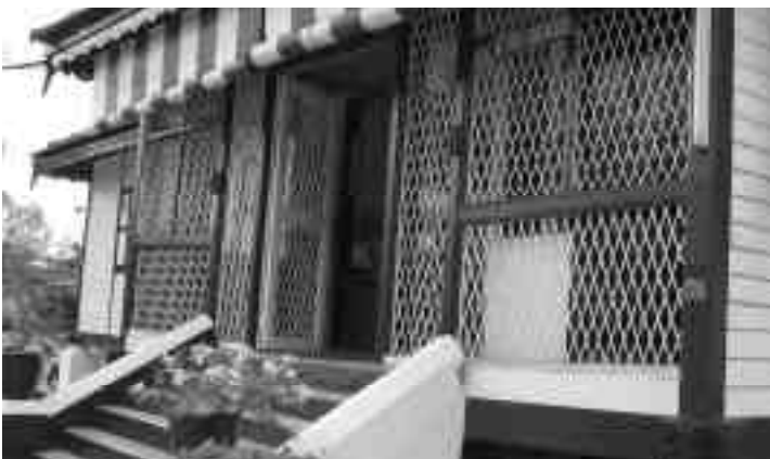
Front entrance, note the ventilation device
