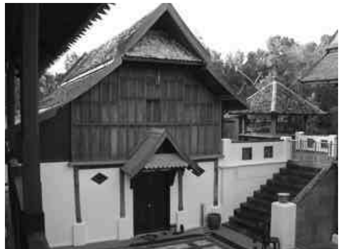
Norhaiza Noordin's home The courtyard, with traditional houses grouped around it.
