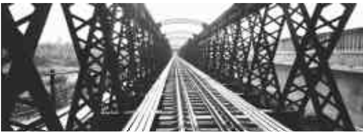
Victoria Bridge, Kuala Kangsar, Perak by Syed Zainal Rashid
