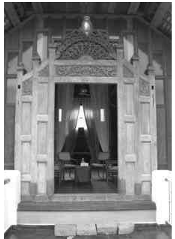
Pintu Gerbang Dato Perdana Norhaiza has placed this 150 year old gateway in a protected position.
