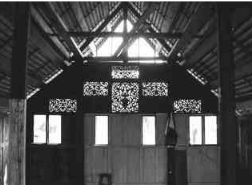
Interior of 2nd house Rear gable end of Rumah Ibu with superbly carved windows. Simple solid shutters close the lower windows.
