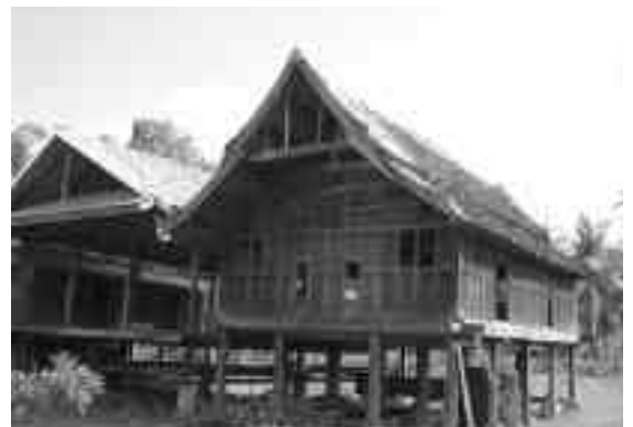
Houses under restoration. Old houses in process of re-erection
