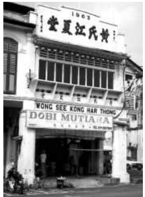
Typical shophouse façade in the town centre. photo: Diana Cooper.
